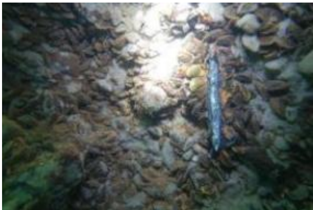
8#墩基础顶面露筋
